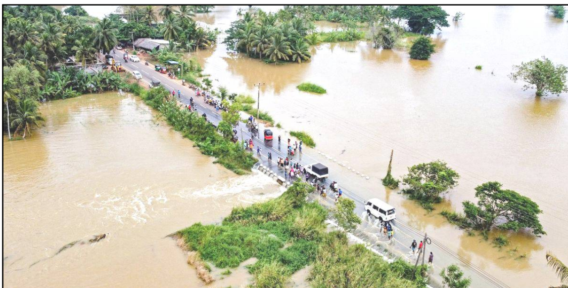
Colombo: November 22 nü nungi tenzüka Sri Lanka nung tzüinglu dak sendakba lendong balala agi nisung 463,000 tema dak kongshiogo, ta linük Disaster Management Center (DMC)-i metetdaksü. Administrative districts 25 nungi 24 nung kibong 138, 191 nungi nisung 463,569 tzümetsüing, süngtong laoba, mopung tesashi aser anentsüh agi kongshir lir ta DMC-isa metetdaksü. DMC-isa, nisung 15 asüba, nisung 20 yiruba aser ka samara bushia aliba metetdaksüogo.
