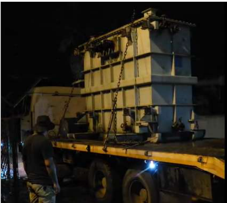
July 12, 2026 aonung Supermarket sub-station-i transformer ka bener arudang agiba noksa ka angur.
