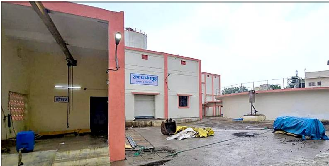
August 24, 2026 nü Nagpur yimti kübok Godhani yimdak water treatment plant ka nung chlorine gas leak asüba sülen tangokba noksa nung angur. Anepongi 1:00 ako nung 900-kg capacity chlorine gas cylinder leak asüba sülen nisung aika hospital-i anir ogo.
