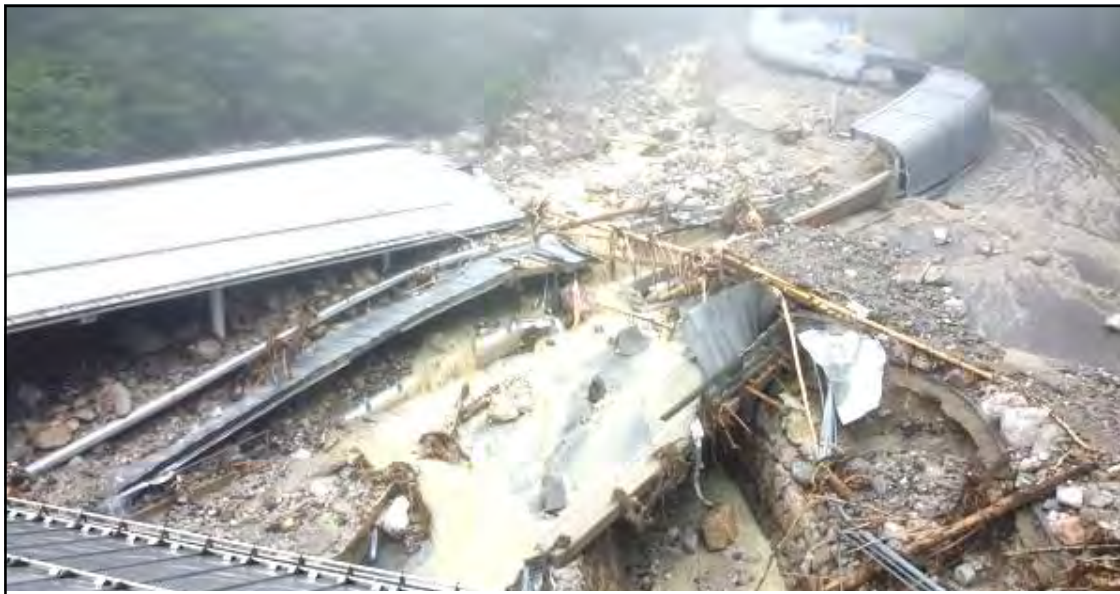
Königssee, Germany nung July 18 aonung yipru tesashi aitba sülen bobsleigh aser luge track ajunga raksar aliba noksa nung angur.
